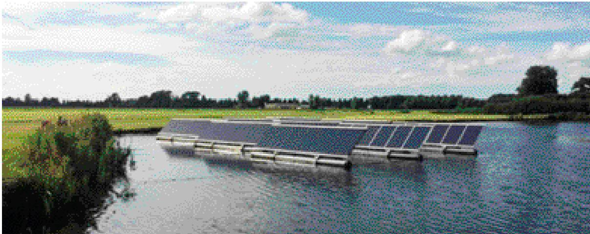
Fig 2 - Floating Solar, ZOGRUNN project (Photo: RVO).
