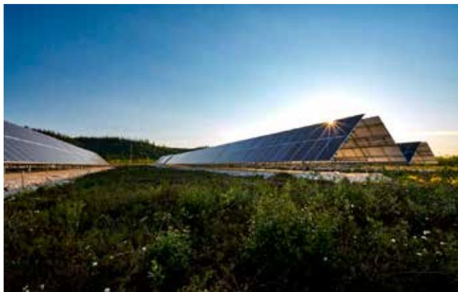
Fig. 1 - The Old Crow Solar Project, a 940 kW system installed by the Vuntut Gwitchin Government in Old Crow, Yukon, 128 km north of the Arctic Circle (Photo: Solvest Inc.).<sup>3</sup>
