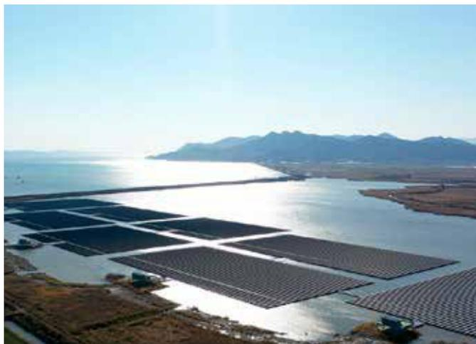
Fig. 3 - 25 MW Floating PV system at Goheung-gun, Jeollanam-do, Korea.
